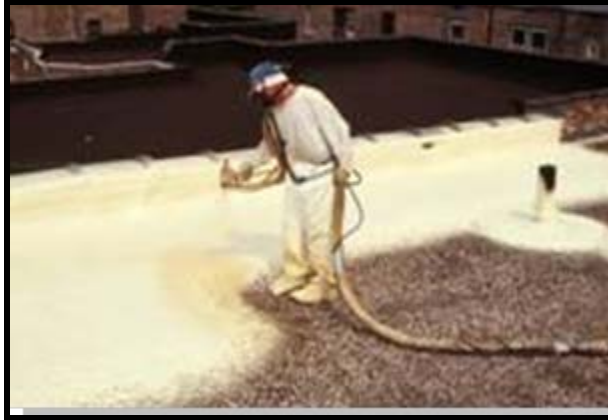
SPF on built-up roofing
