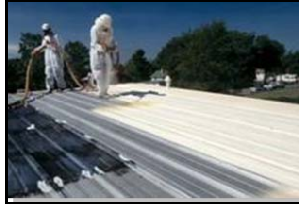
SPF on metal roofing
