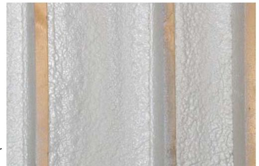
qualities, moisture vapor retarder and air barrier that closed cell foam provides. Much more than just insulation, SPF offers improved building durability, healthy indoor air quality and enhanced moisture management — all critical factors in building quality homes.
