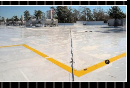
The following roofing system components were installed over the existing roof deck, which is a 2.5-inch lightweight concrete over 24-gauge steel form decking:
