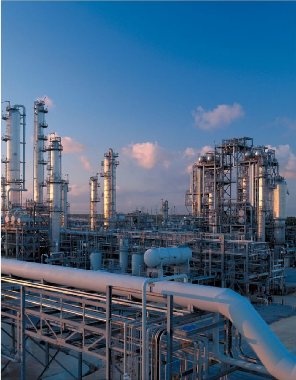
Port Neches, Texas Propylene Oxide Facility
