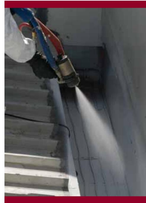
These specialty amines generally possess soft, flexible polyoxypropylene backbones that significantly contribute to the hydrophobic/waterproof nature of the respective polyurea coatings. These alternating hard block/soft block polymer units are linked by DETDA, which is commonly referred to as the "chain extender" of the system.
