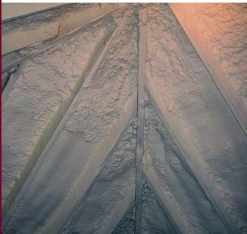
Unvented attic assembly with intumescent coating ignition barrier.
